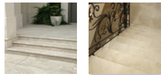
steps and risers
